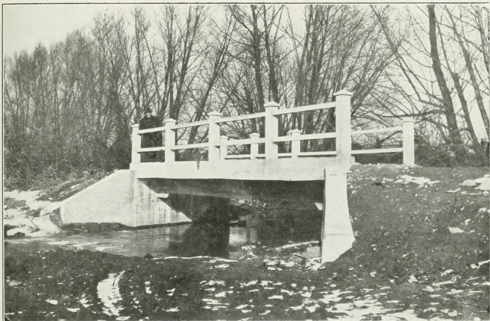
A Reinforced Concrete Bridge with Concrete Railing. In Markham Township, County of York.
